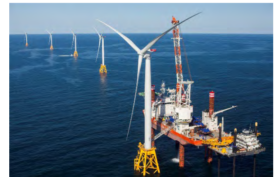
Heavy lift installation vessel
